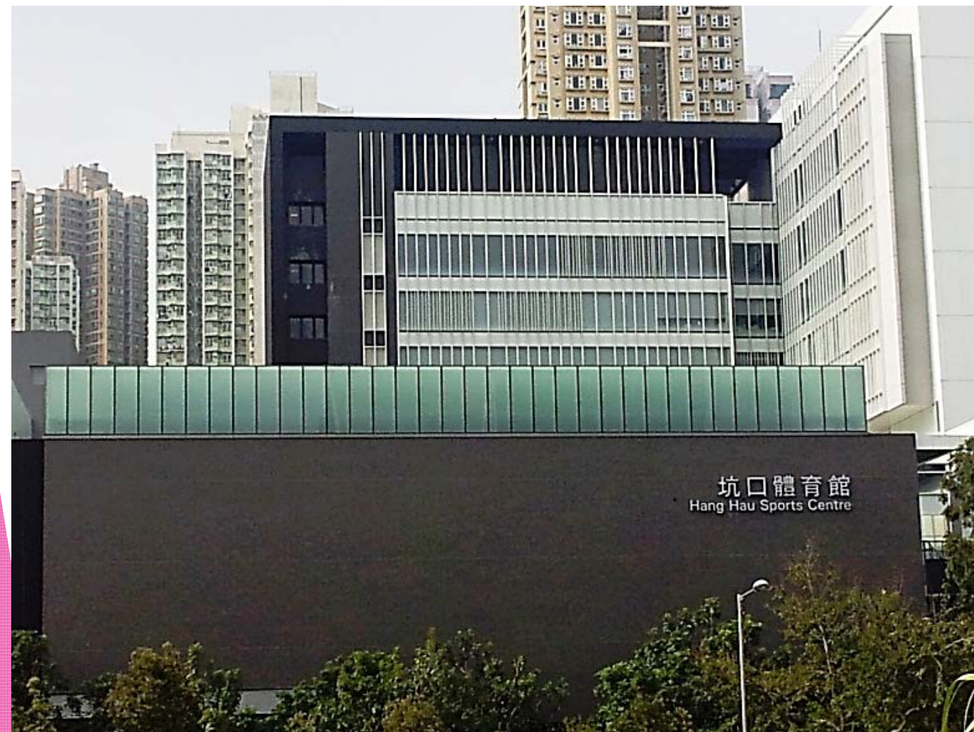
Fire Resistant Glass Works & Structural Skylight Works
