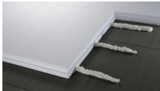
... place the insulation board and press home – that's all.
