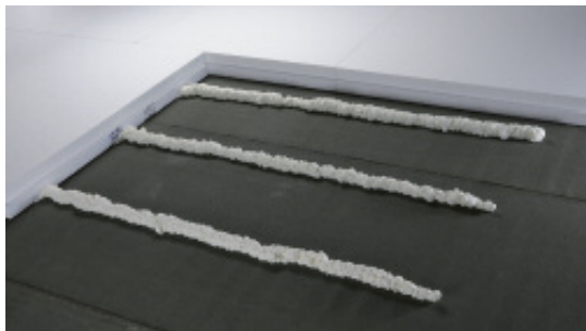
Apply the adhesive beads, ...
