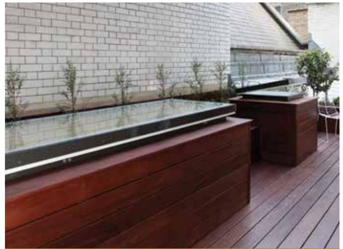
Em-Glaze Modular to builder's upstand
