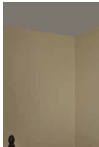
Before Em-Tube installation
