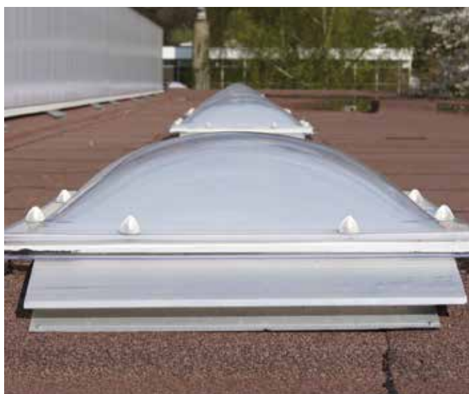
Em-Dome ECO on Em-Curb ECO PVC 350mm upstand
