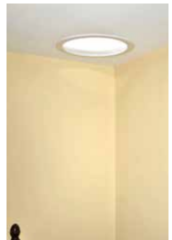
After Em-Tube installation
