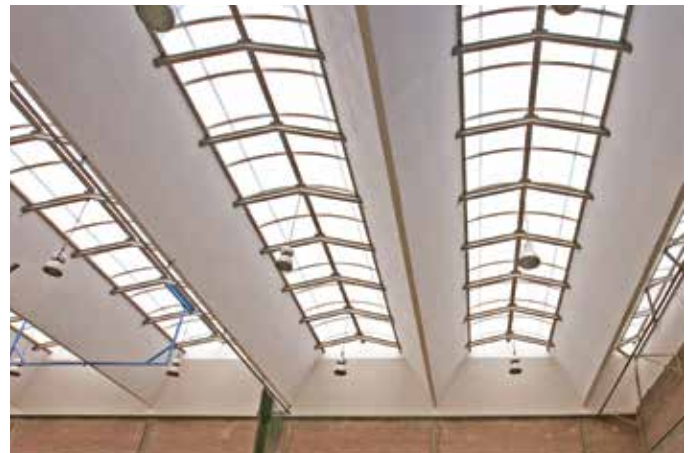
Em-Vault in opal diffused with multiwall glazing
