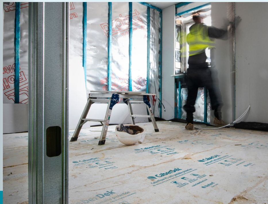
CaberDek is perfect for situations where flooring is laid before the building is weather tight and whilst there is still likelihood of construction mess.
