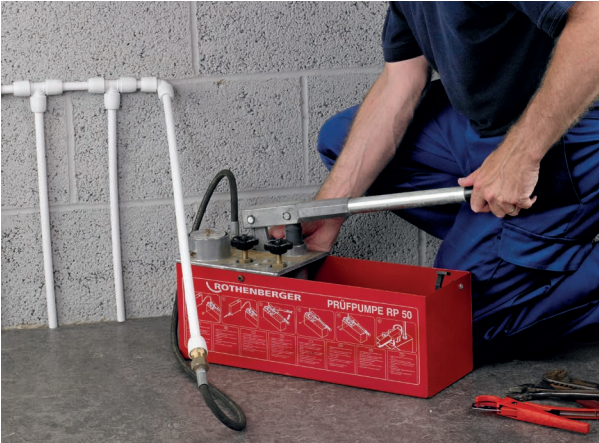
Fig. 60 Pressure testing
