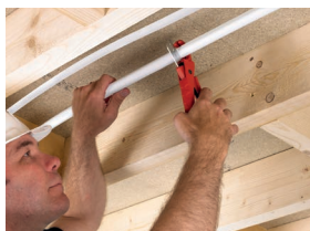
Measure and cut in-situ
