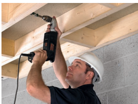
Fig. 31 Hep 2 O speeds up installations because pipework can be easily cabled through drilled joists
