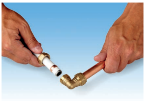
Ensure pipe is fully inserted
