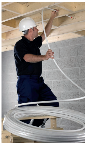
Fig. 22 Packaging retains pipe until last metre
