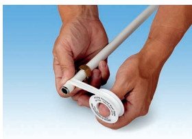
Apply PTFE tape if required
