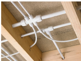
Fig. 31 Hep 2 O speeds up installations because pipework can be easily cabled through drilled joists
