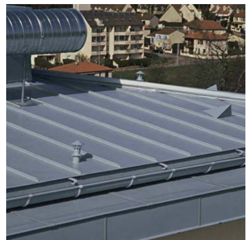
Air inlets and outlets are generally linear (at least 10mm wide) but can be individual (see photo). The ventilation must correspond to BS 5250: 2002.
