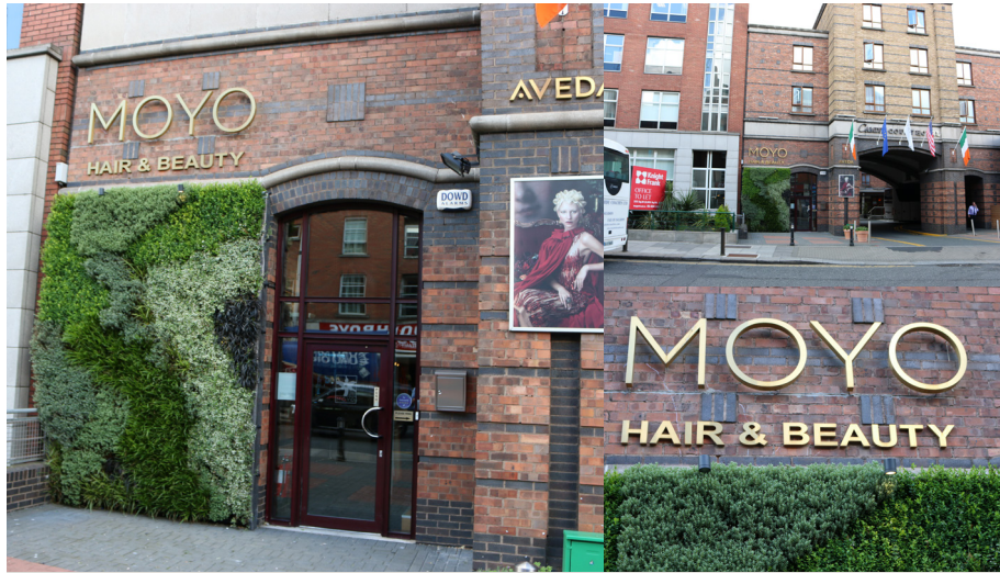
This ANS Living Wall was installed at the Aveda - Moyo hair salon in Dublin and the owner enjoyed a 30% increase in sales the following year
