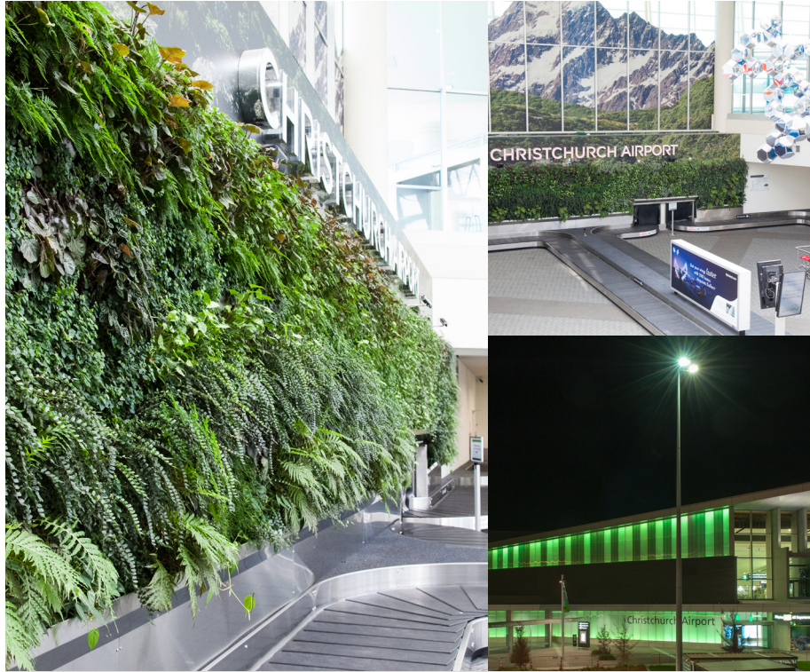
This ANS Living Wall was installed in the noisy baggage reclaim area at Christchurch Airport to reduce noise levels.
