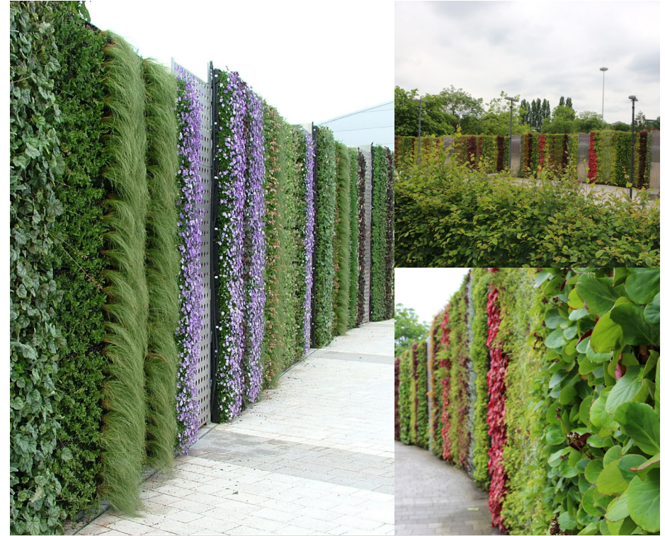
Likewise, this ANS Living Wall was installed at the NEC exhibition centre as a sound barrier to deaden noise from the arena.
