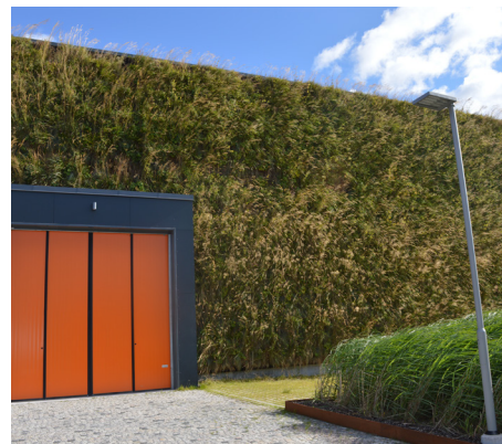
Ursvik Recycling centre in Sweden has been successfully installed for years and proves that the ANS system can cope with the cold.
