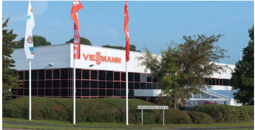
Viessmann UK headquarters, Telford
