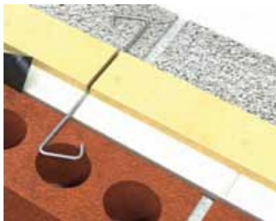
Fig 1 Wall tie sloping outward. Sloping wall tie in preformed slot.
