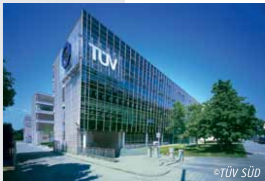
TROX air handling units are regularly examined (e.g. by TÜV SÜD, Germany)
