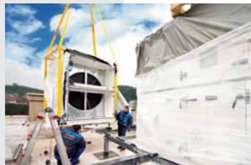
Delivery and installation of a weatherproof X-CUBE
