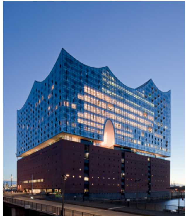
Elbphilharmonie Hamburg: TROX ventilation and air conditioning in all concert halls
