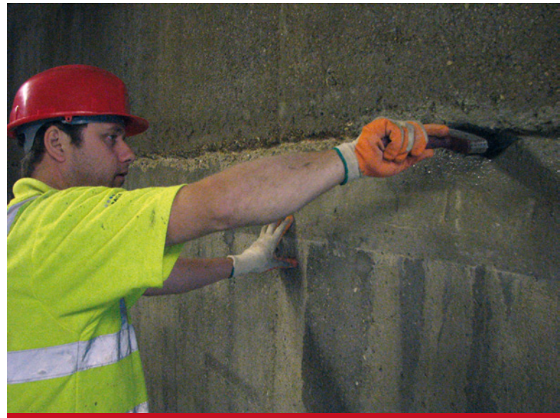
Triton TT Super can also be used in the repair of construction joints
