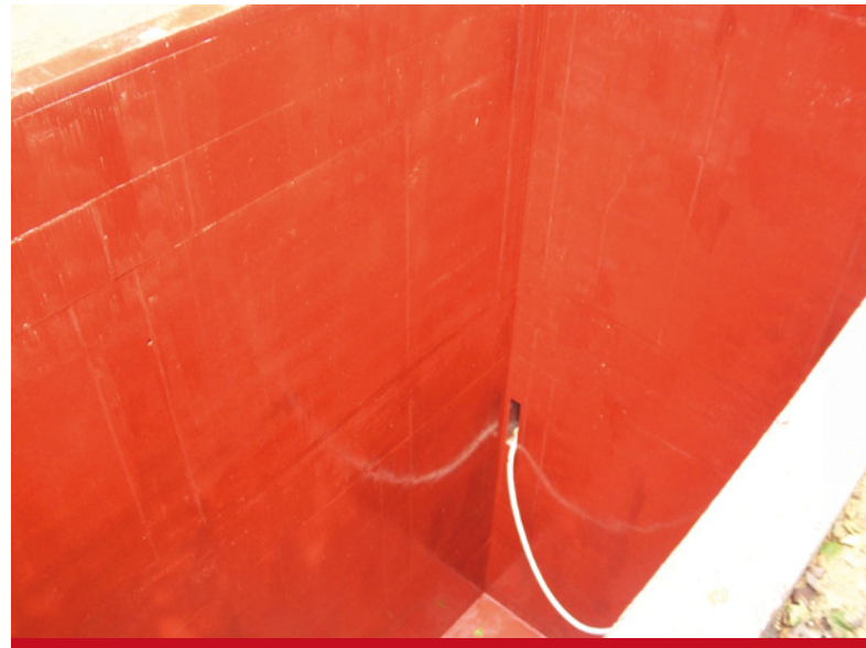
Tri-Seal used as a surface applied waterproofer to car lift shaft
