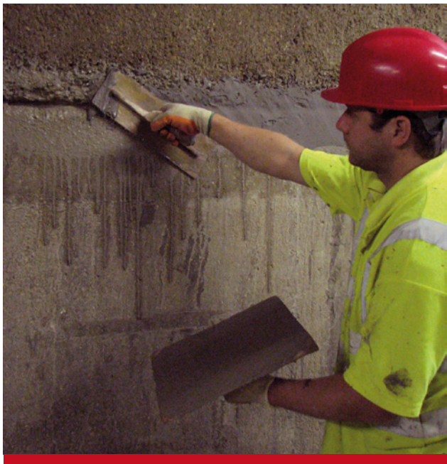
Construction joint repair using Triton Fillet Seal.
