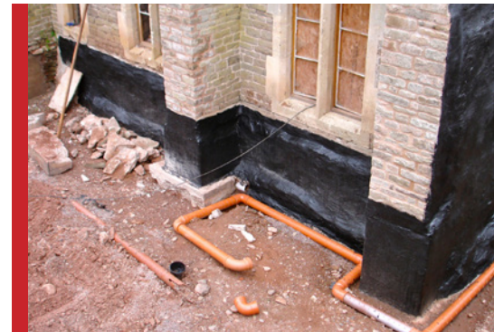
TT Vapour Membrane used as a landfill gas barrier and applied to external walls below internal floor level to the base of the wall/foundation level and internally to new floor slab.
