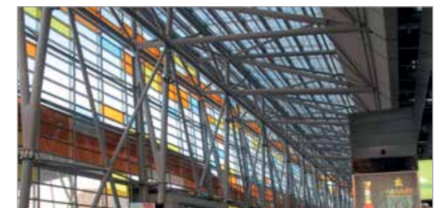
| Trimo Steel Construction
