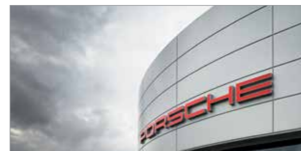
| Qbiss One, Metal Modular Façade System
