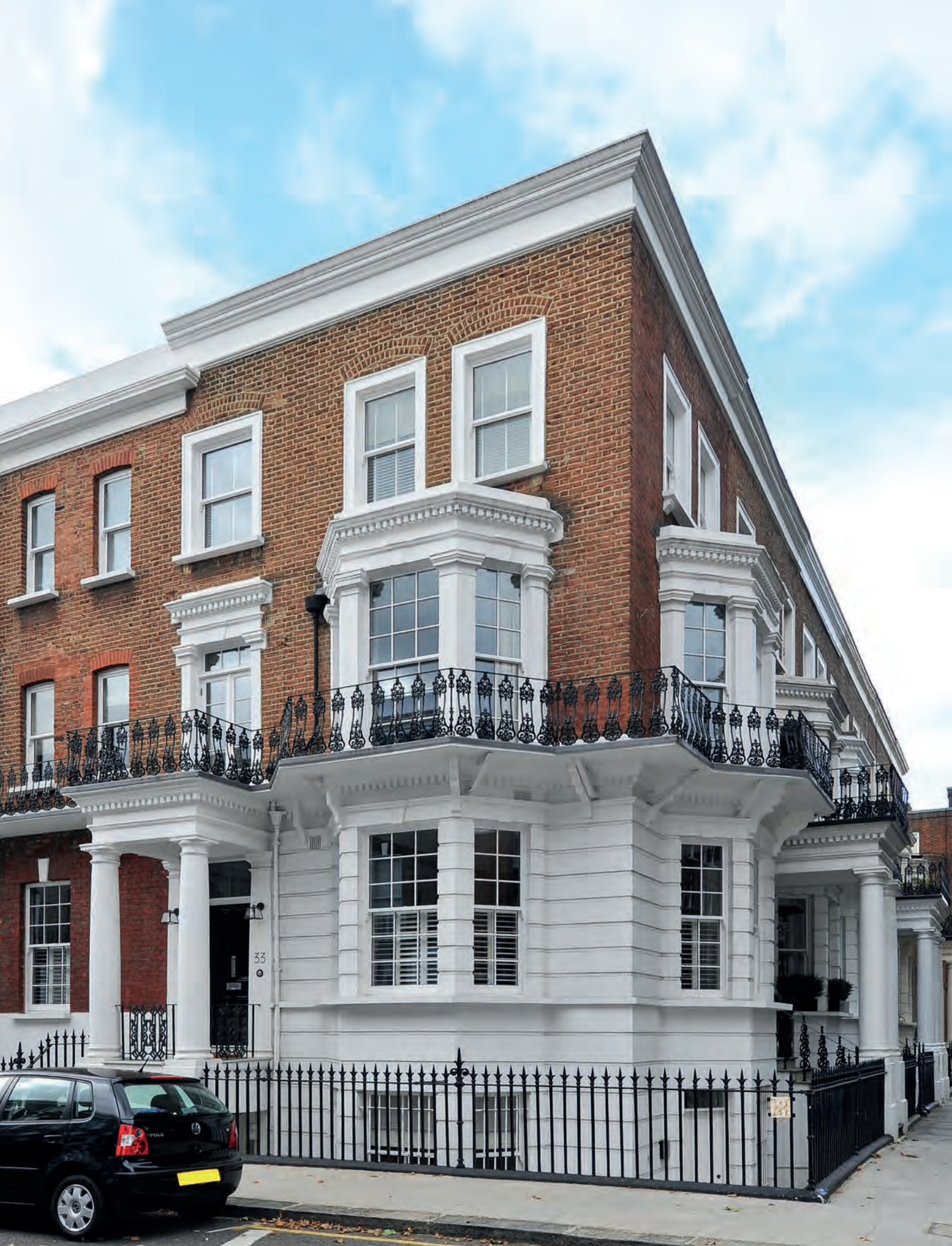
Complete new sash windows manufactured and installed.
