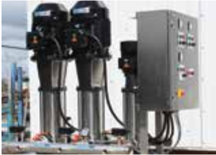
FIXED SPEED BOOSTER SET WITH JOCKEY PUMP
