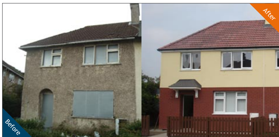
Boswell properties refurbished by Liverpool Mutual Homes using Structural External Wall Insulation.
