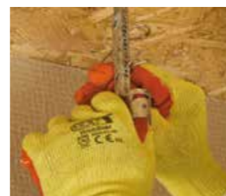
Sto Nonius hangers installed using a laser levelling device.
