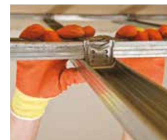
Sto primary & secondary channels installed.
