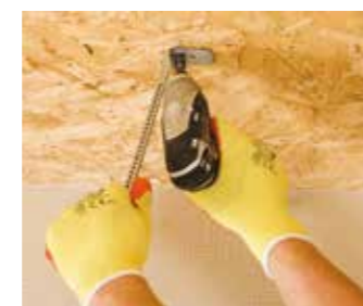
Sto strip hangers fixed to substrate using suitable fixings.
