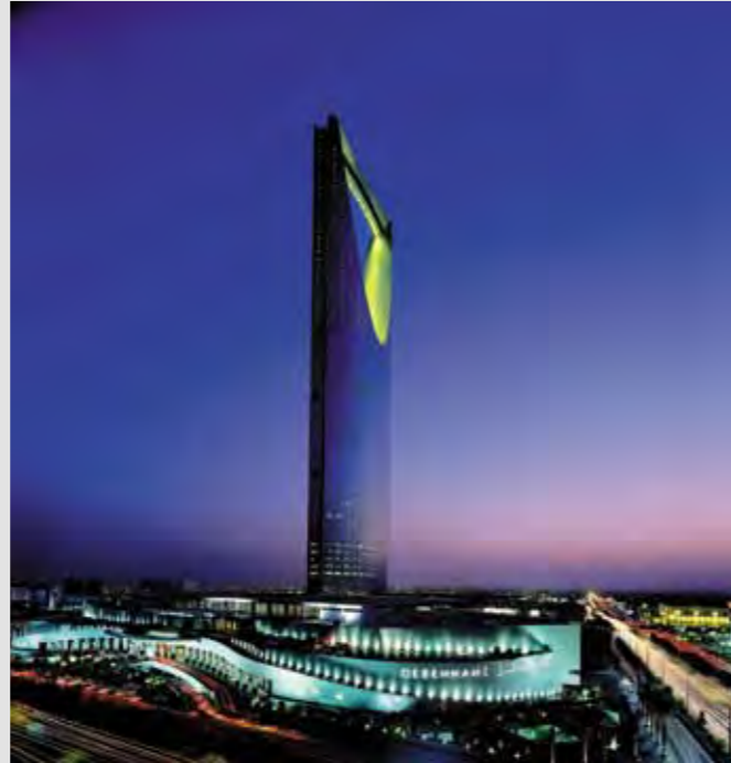
Kingdom Tower, Riyad, Saudia Arabia
