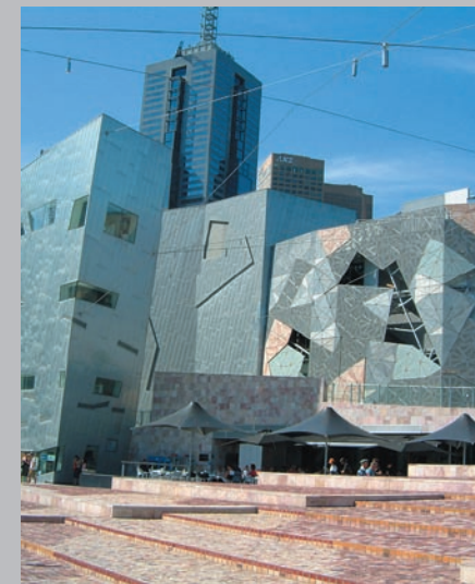
Conference Square Commercial Building Sydney, Australia
