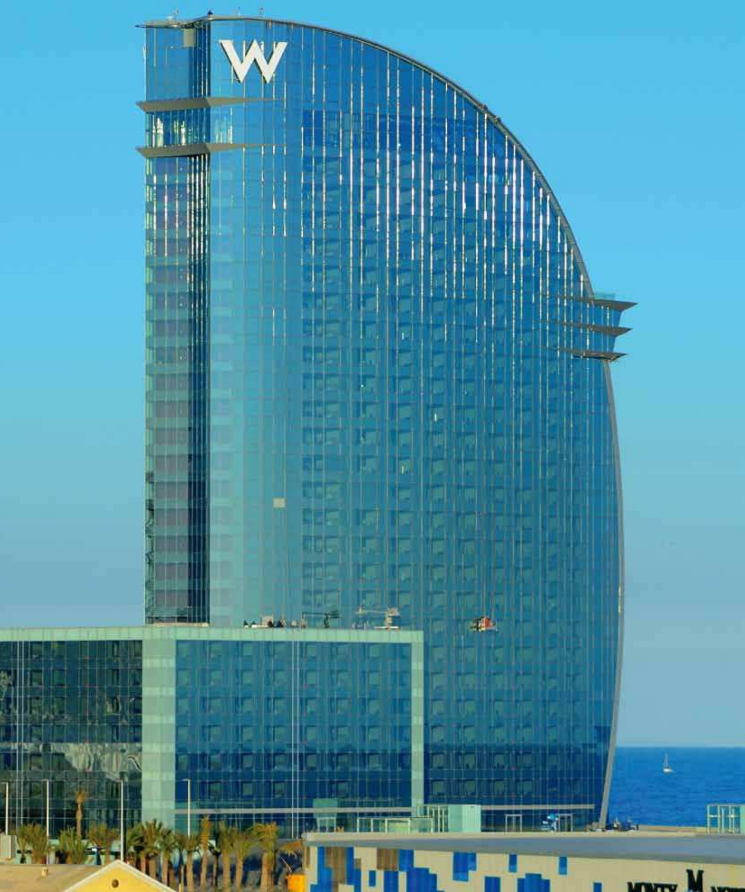
Hotel Vela, Barcelona, Spain This impressive façade of the new hotel Vela was entirely bonded and sealed with Sika's structural glazing weatherproofing products.
