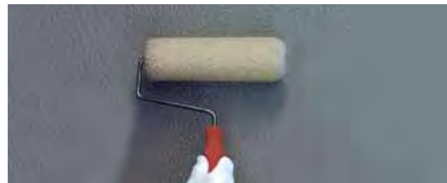
Application of Sikafloor®-264 Thixo high build coating with a textured roller.
