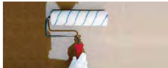
Primer application with medium pile roller.
