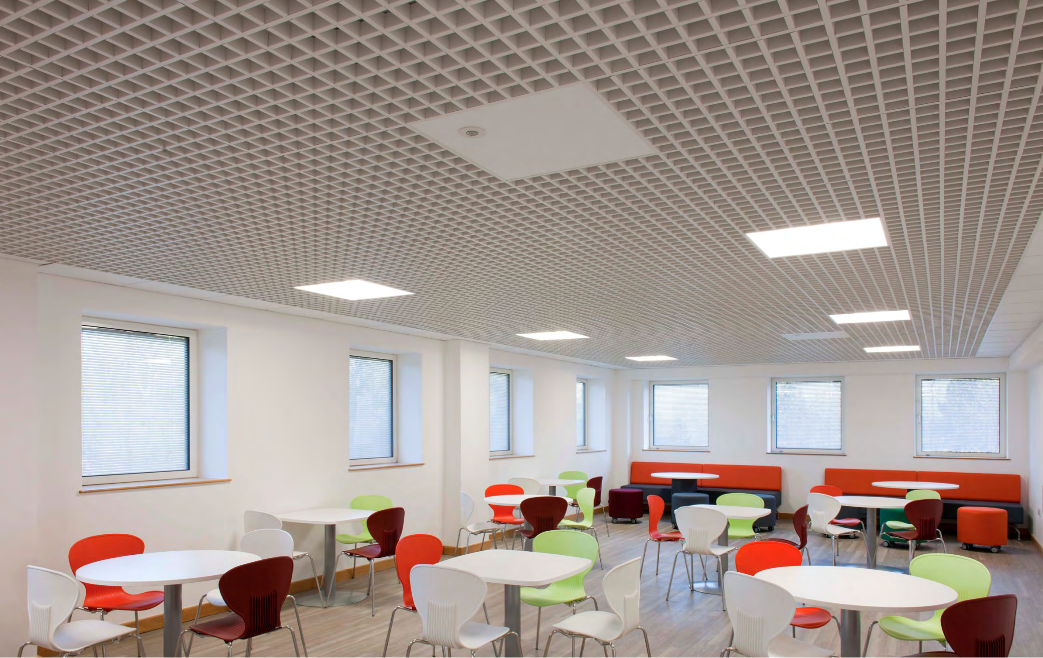
Trucell – Kent County Council
