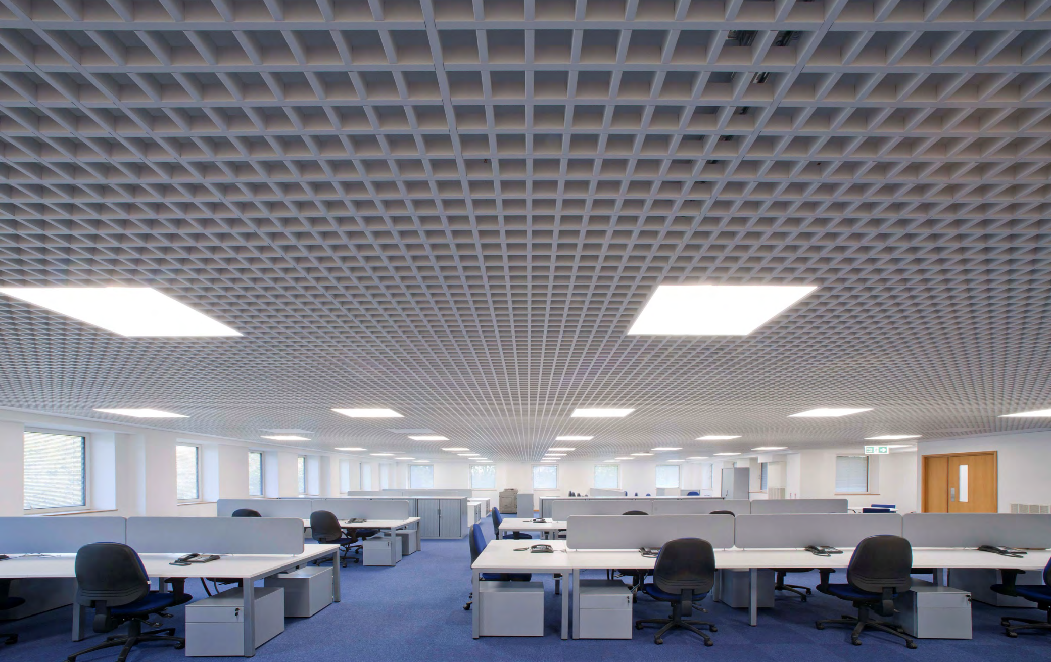
Trucell – Kent County Council
