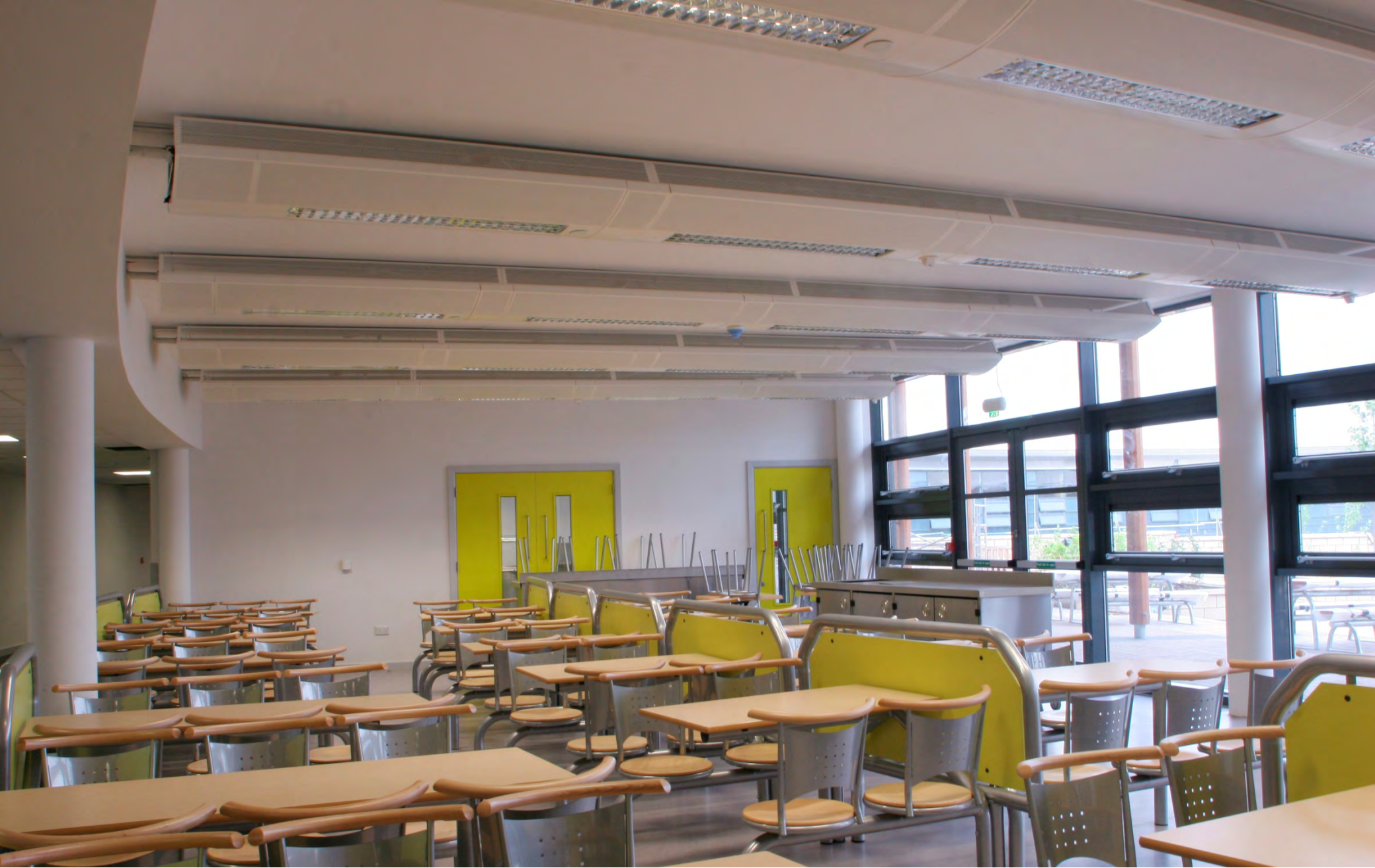
System 600 – Hadley Community Learning, Telford
