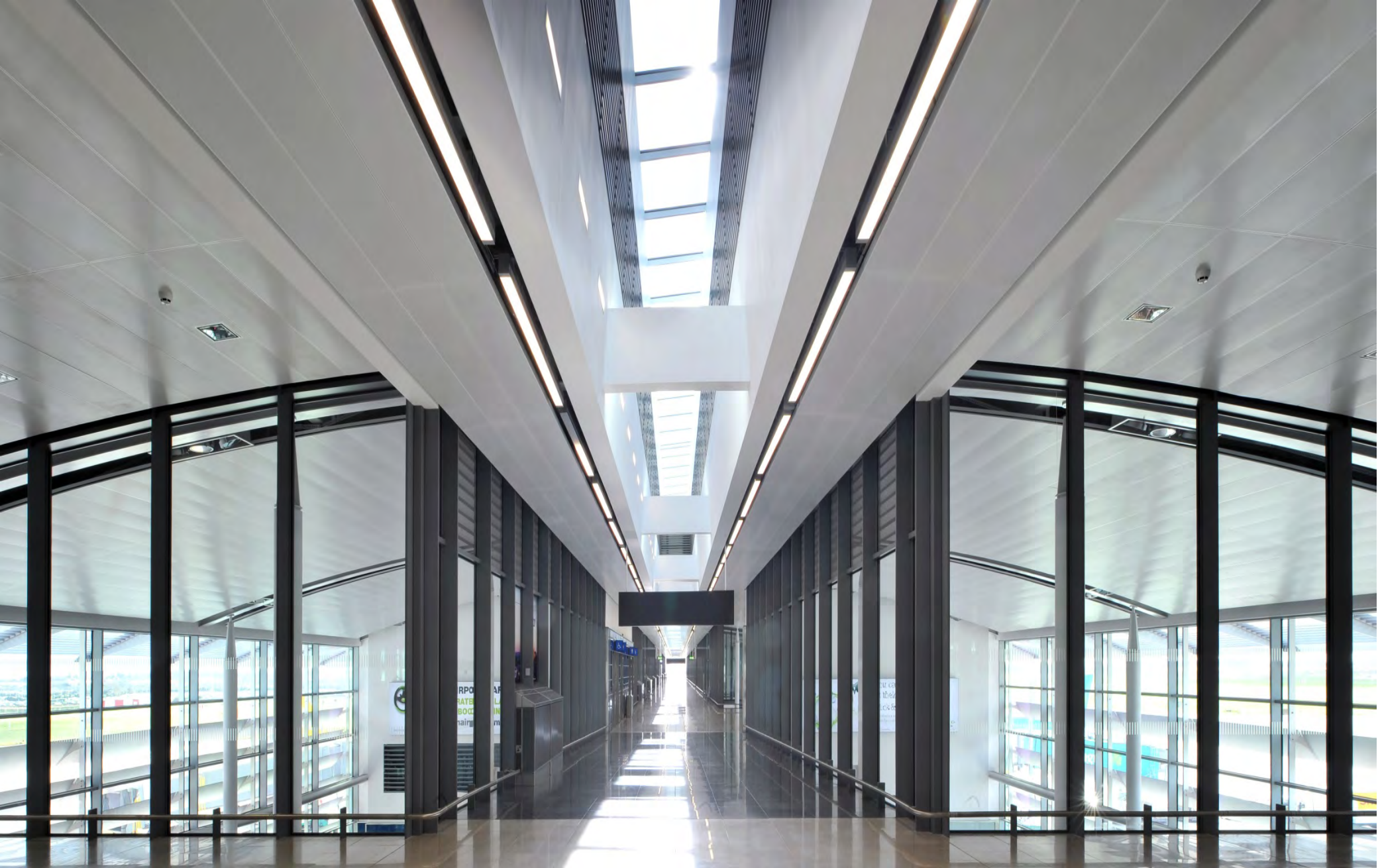
System 200 – Terminal 2, Dublin Airport
