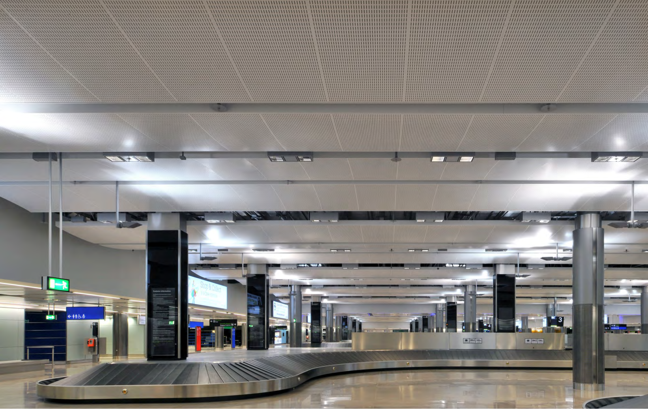
System 205 – Terminal 2, Dublin Airport
