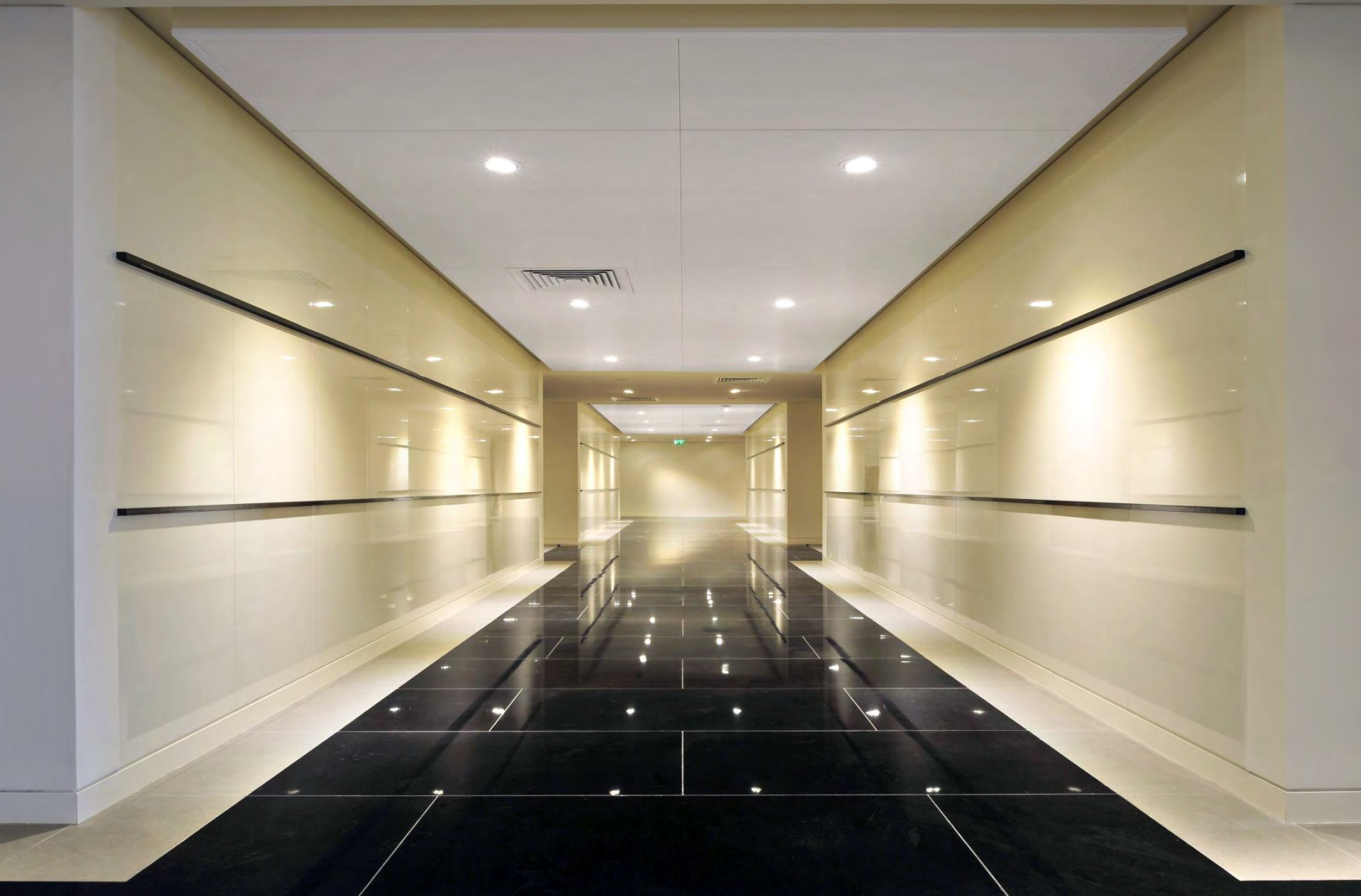
System 150 – International Tower, Abu Dhabi
