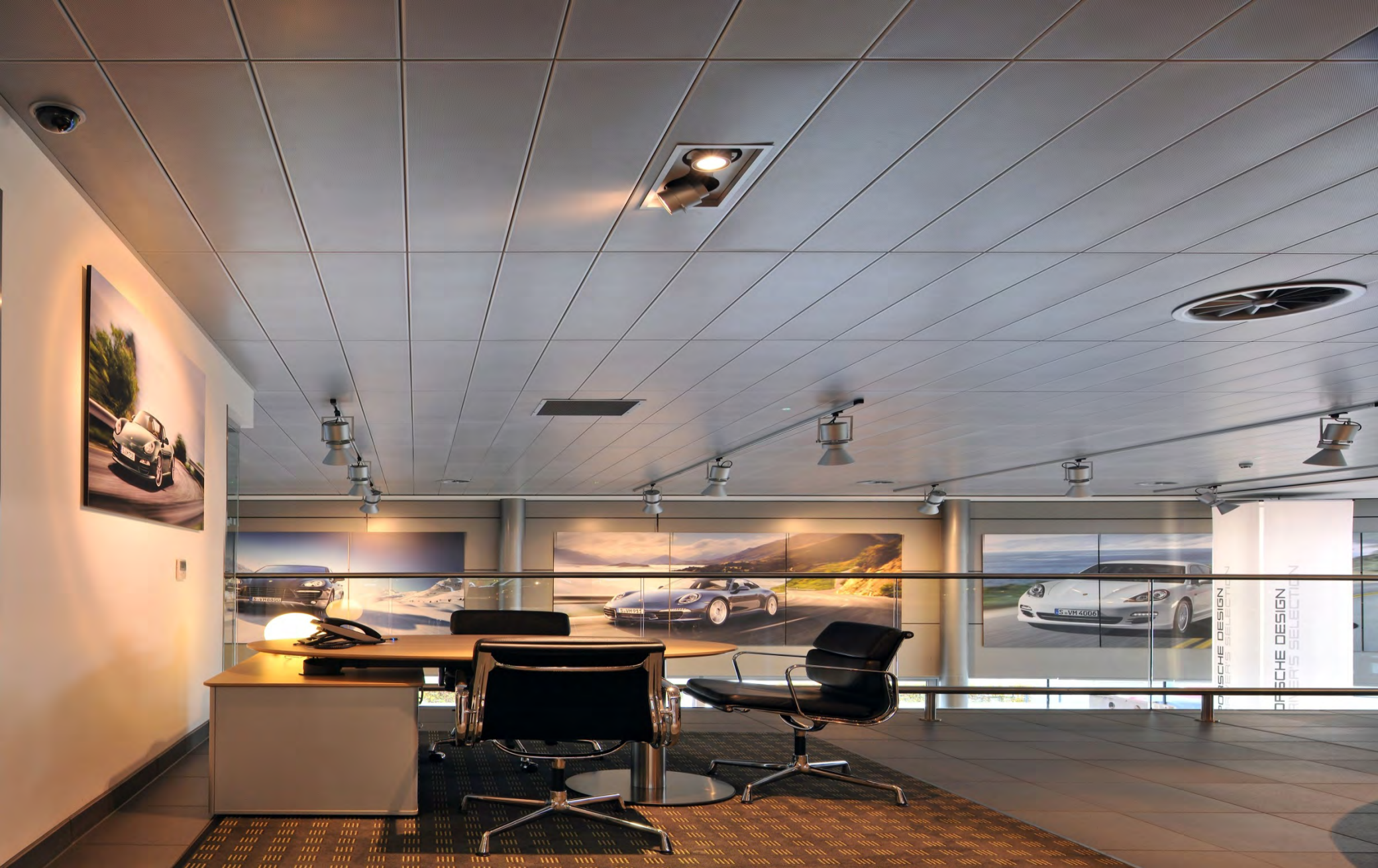
System 120 – Porsche Centre Solihull
