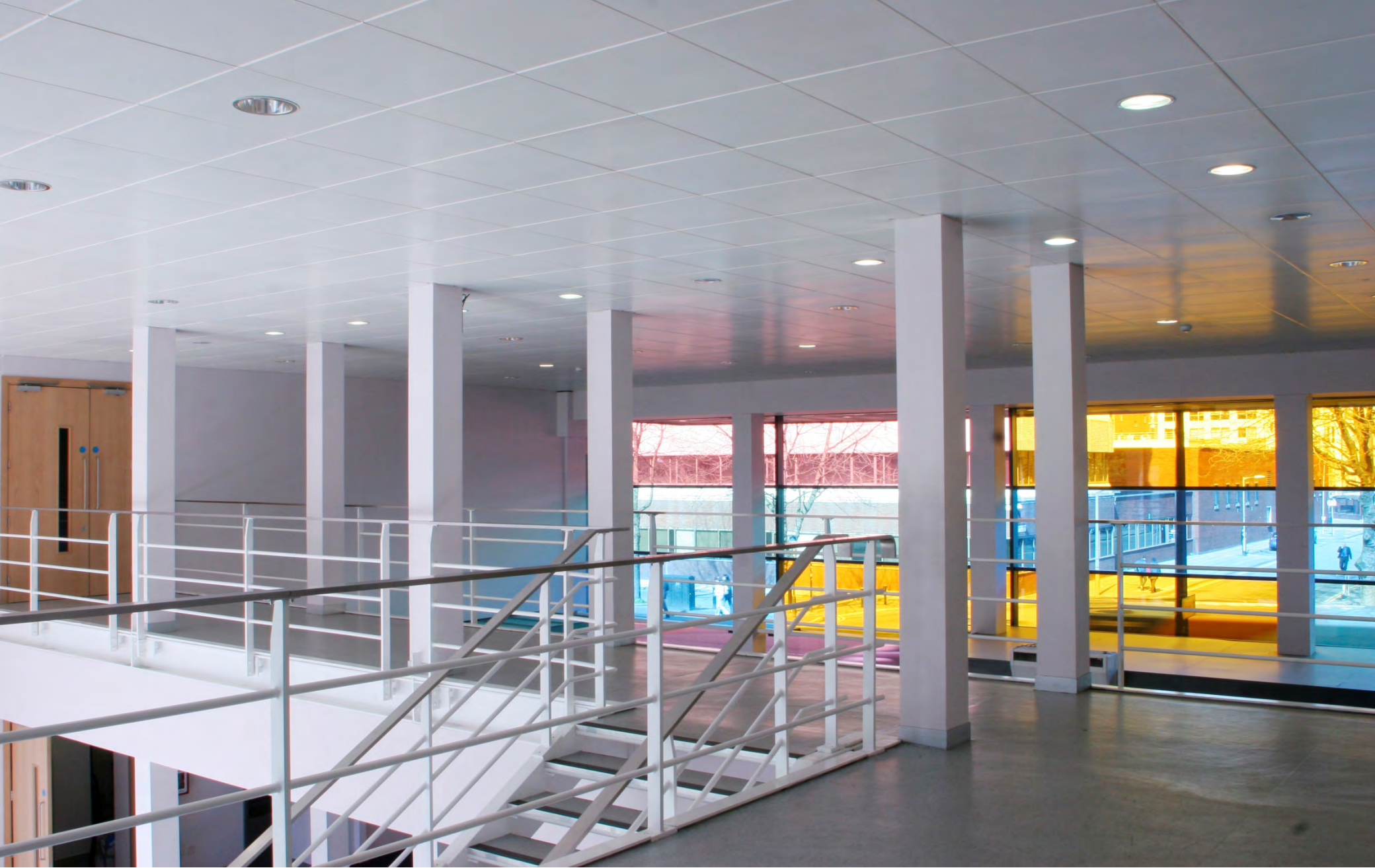
System 120 Plank – Manchester Metropolitan University
