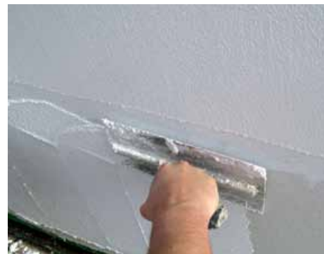
■ Top Coat Application
