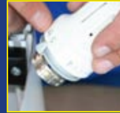
10. Mounting of the thermostatic head
