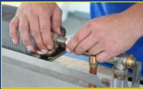
7. Mounting of the adjusting screw coupling
