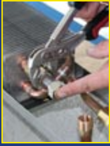
7. Mounting of the adjusting screw coupling
