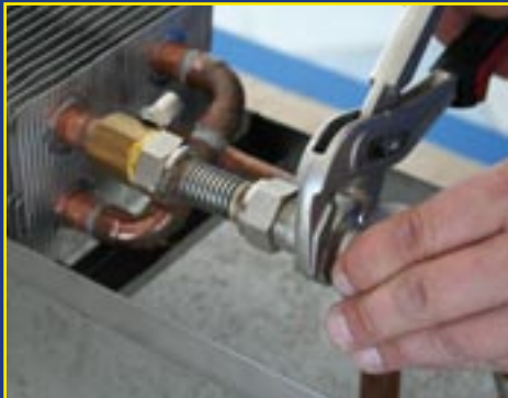
10. Mounting of the thermostatic head
