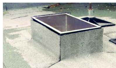
2. Waterproof the base and upstand.
