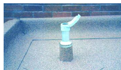
2. Waterproof the base and upstand.
