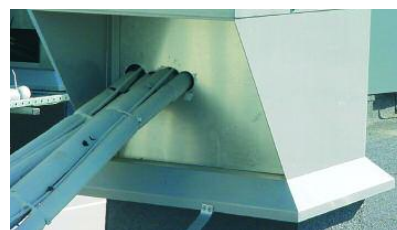
4. Cut pull-out panel to pipe work.
