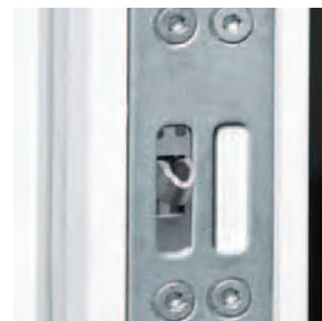
4. Hook bolts in hardened steel combined with a reinforced front plate can resist even severe attacks from the burglars' tools.
