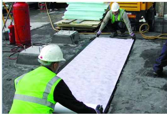
Install reinforcement layer.
