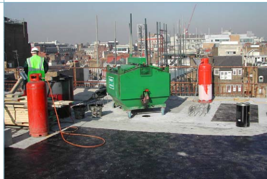
Apply Radmat Surface Conditioner.
