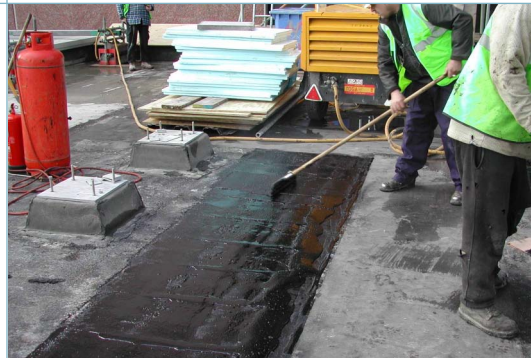
Apply in 1m wide bays.
