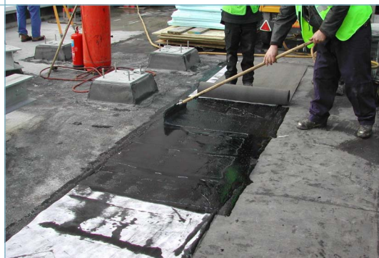
Install final layer with protection sheet.
