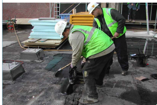
Install first layer.
