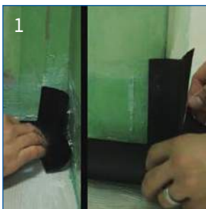
1 Fit the floormitres in internal and external corners
