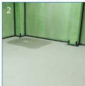
2 Fit the Cove former (QCF35) on floor and internal verticals. Use EFA75 for external verticals if required.
