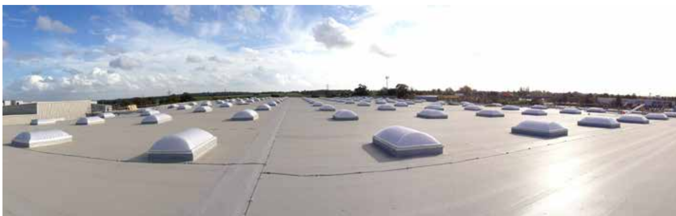
Image of a near-completion roof system with prefabricated sheets in UK
