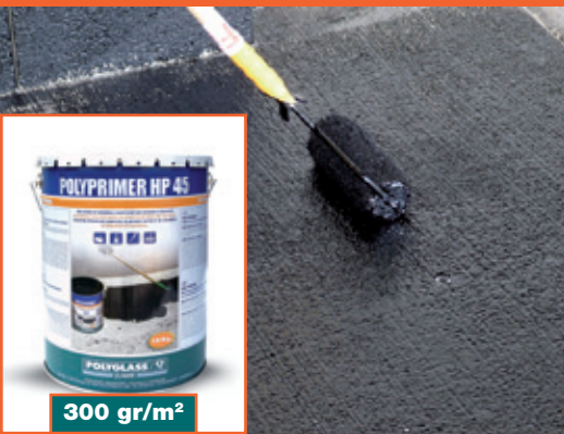
1 - Treat the area to be waterproofed with bituminous primer (POLYPRIMER HP 45 Professional).
