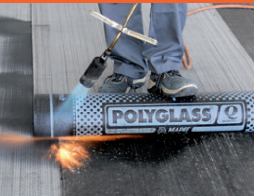
7 - Apply the second sheet with adequate overlapping.
