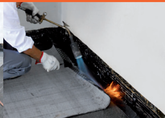
6 - Pull the sheet up to a certain height against vertical surfaces.
