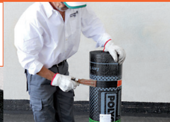
3 - Completely strip away the product identification tape.
