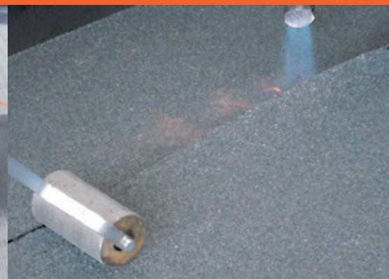
9 - Roll the overlapping areas using the special pressing roller.
