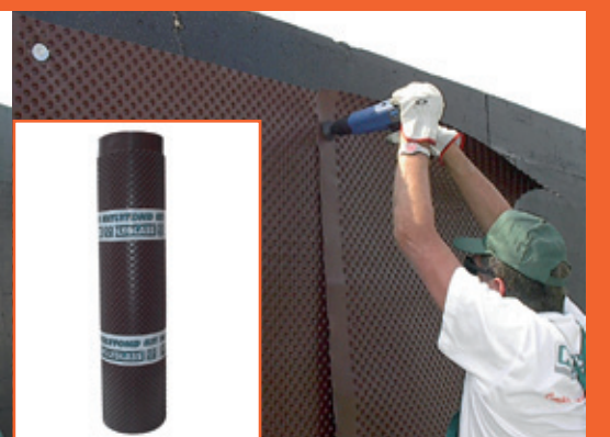
11/12 - Apply mechanical protection (e.g. POLYFOND KIT membrane in embossed HDPE) over the waterproofing membrane if necessary.
