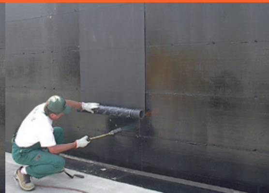
5/6 - Apply the membrane sheet by first fastening the upper part on the wall and then proceeding downwards.
