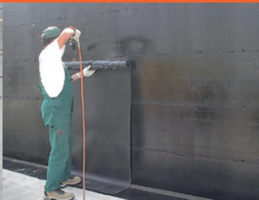
5/6 - Apply the membrane sheet by first fastening the upper part on the wall and then proceeding downwards.
