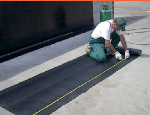
4 - Cut the membrane sheet to the size of the surface to be waterproofed.
