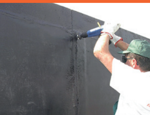
10 - Fasten the bituminous membrane to the wall using the appropriate mechanical fastening systems at the overlapping points.
