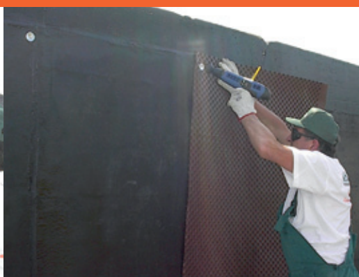
11/12 - Apply mechanical protection (e.g. POLYFOND KIT membrane in embossed HDPE) over the waterproofing membrane if necessary.
