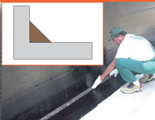
2 - Position the corner border at the base of the wall to be waterproofed.
