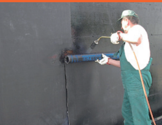
7 - Apply the next sheets by respecting the overlapping points.
