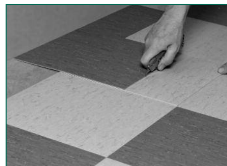
Figure 12 Measuring using an overlapping tile
