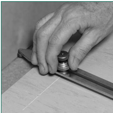
Figure 2 Scribing the wall profile
