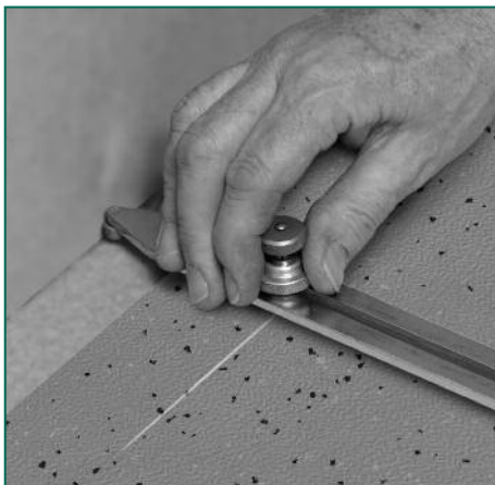
Figure 17 Scribing the wall profile
