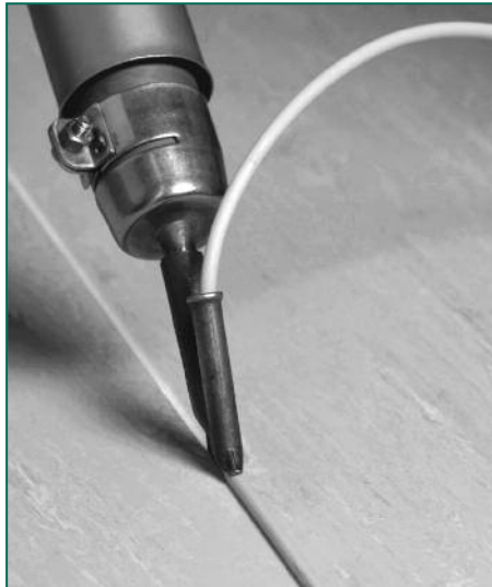
Figure 29 Applying the weld
