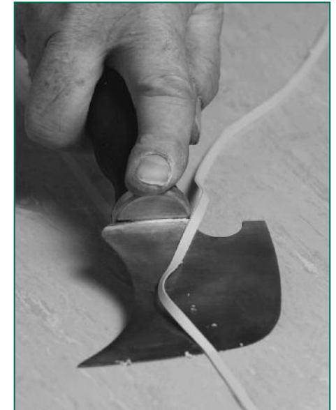
Figure 32 Final trim after the weld has cooled
