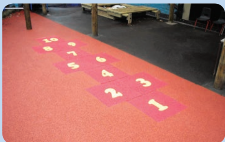
Wetpour Overlay Tarmac - For high level equipment
