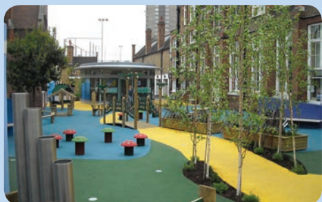
Wetpour Overlay Tarmac - For low level equipment
