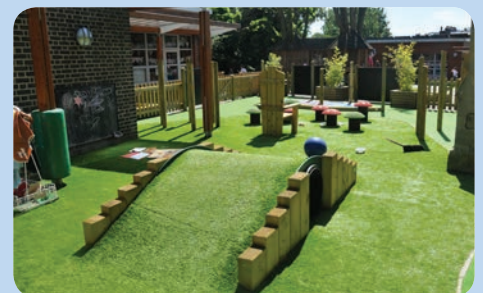
Play Lawn Safer Impact - Recycled foam shock pad on top of 50mm stone & geo textile membrane
