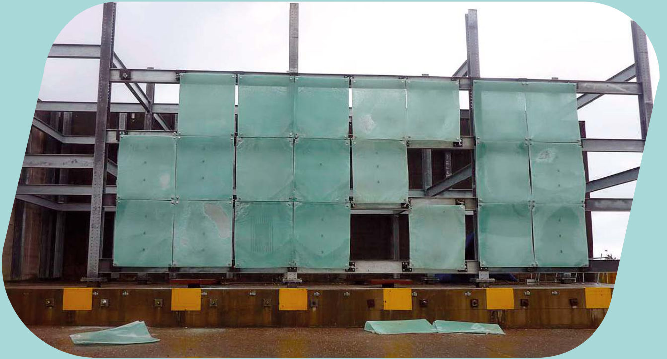
After Blast test.
