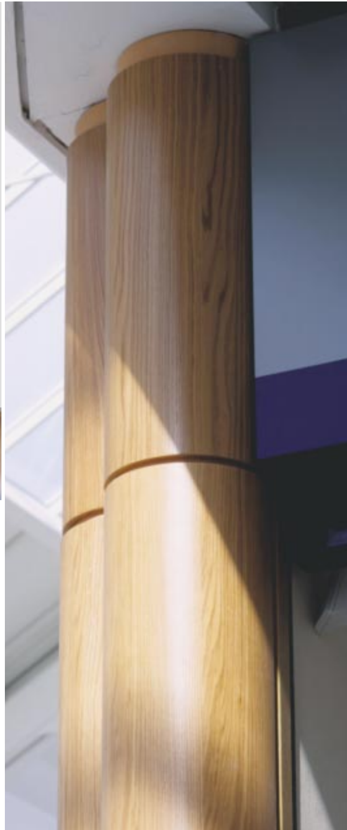
Pendock plywood column casings. Kingsgate Shopping Centre
