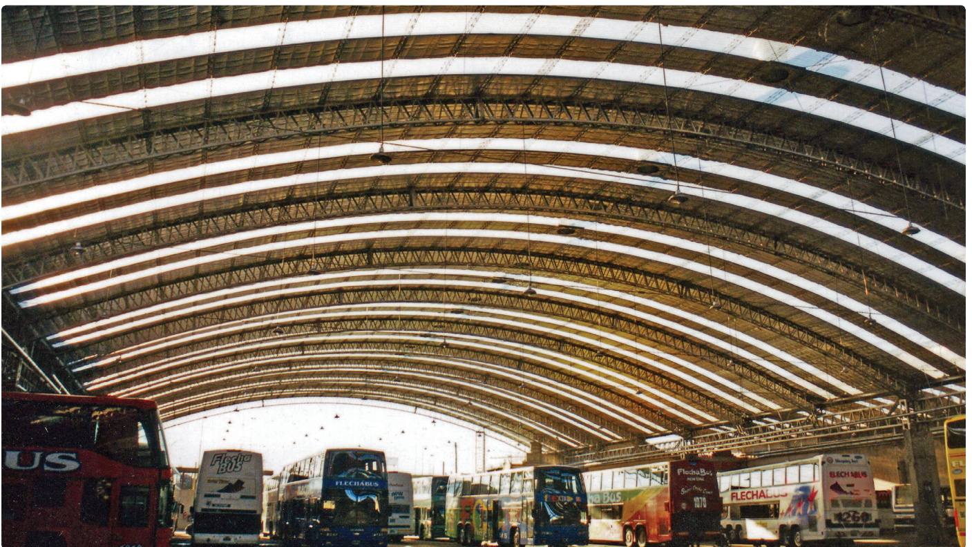
Central Bus Station - Argentina | Bus garage | SUNTUF® Rooflights fitted into a curved metal roof
