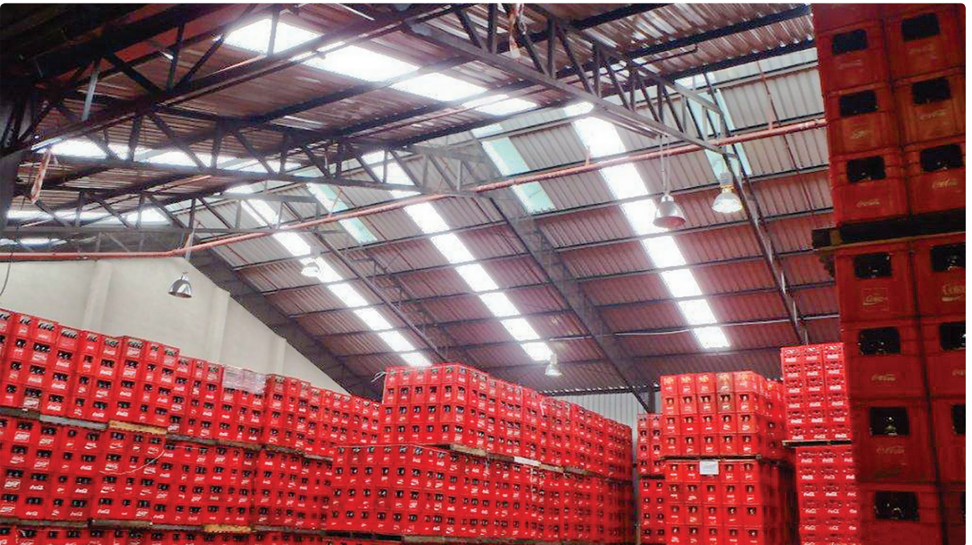
Coca Cola Center - George, South Africa | Industrial warehouse | SUNTUF® Rooflights fitted into a PALRUF® White Opaque 2mm roof
