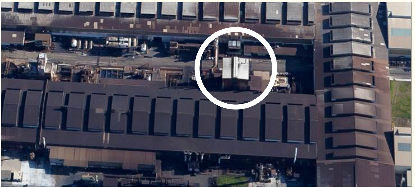
The building in the center is covered with Palruf while buildings around it are covered with metal.
