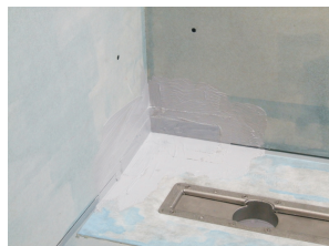
OTL 028 internal corner
