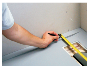
3. With the waste support attached to the tray, measure and cut off the excess material from the wall edge of the tray, to obtain a flush finish from the inside edge of the tray to the finished wall surface.
