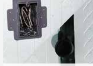
Install electrical, plumbing & roof
