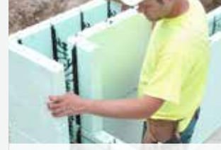
Stack forms & create openings
