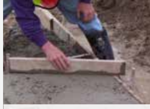
Prepare footings for block
