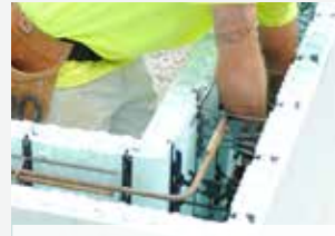
Place rebar in the walls
