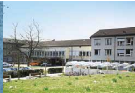
Stair area • Hospital Stadtspital Waid • Zurich • Switzerland
